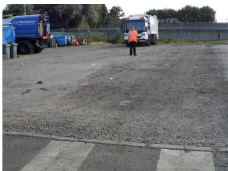
Before the re-surfacing.
